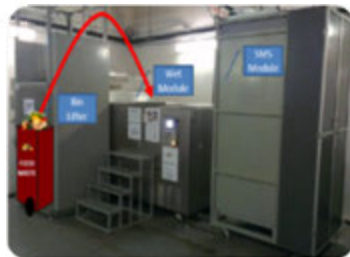
Eco-Wiz Wet system (ecoDigester)
