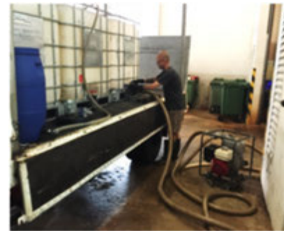
Transferring of slurry to be transported off-site for processing
