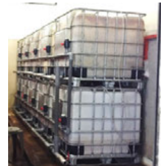
Food waste slurry stored in tanks at bin centre
